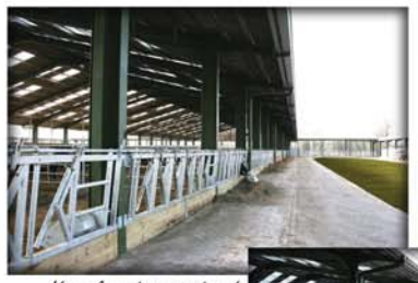
View along the east edge of cubicle building no. 1
