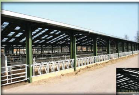
Cubicle 2, self locking yokes
