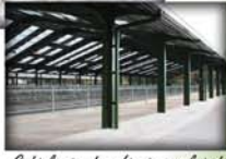
Cubicle 1 when first completed
