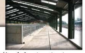
View looking down the edge scraper passage of cubicle 2
