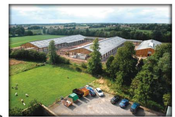
Dairy complex during construction
