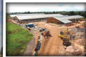
The dairy complex during construction
