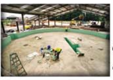
Construction of the rotary parlour
